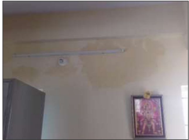
2. Issue of seepage and inconvenient location of electrical switches in BBMP West office
