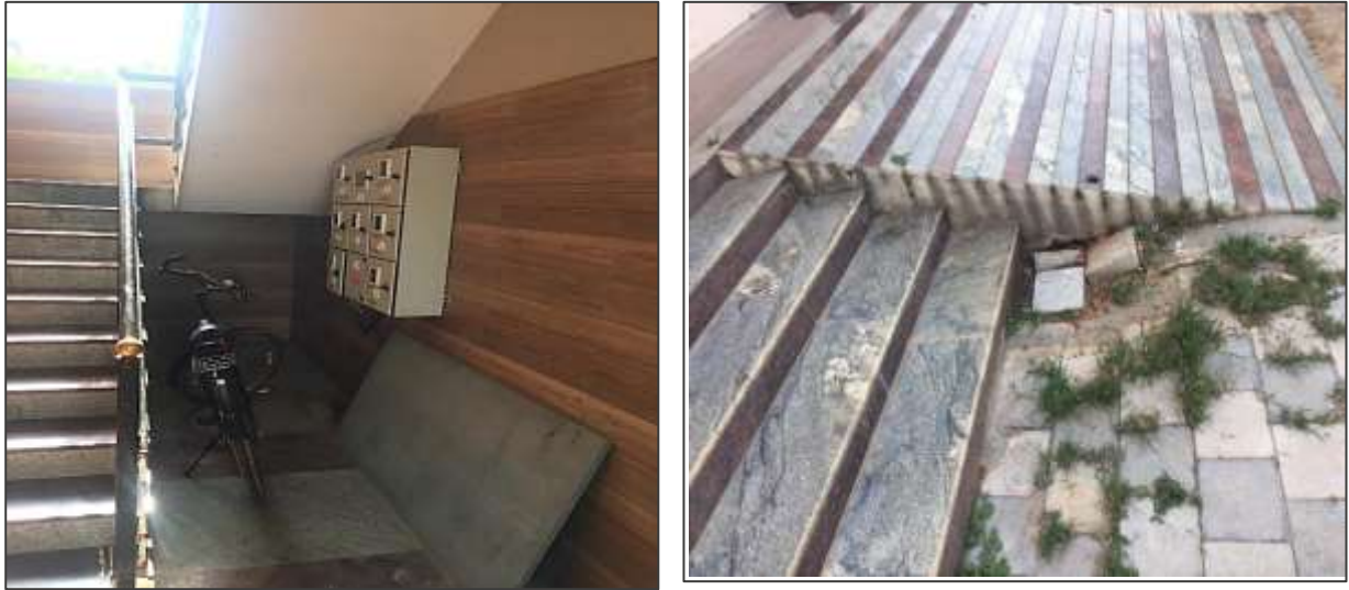
Figure 36: Presence of stairs with railings and ramps
