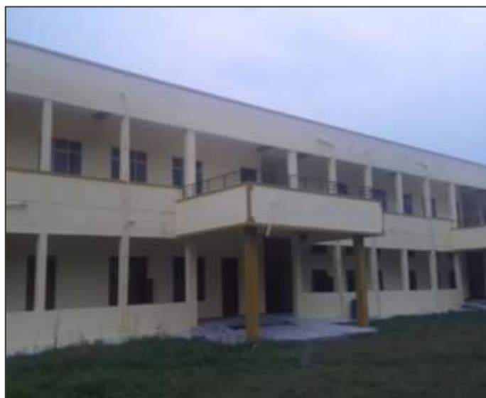
2. Laboratory building for Moodigere Tau Government College, Chikkamagaluru District
