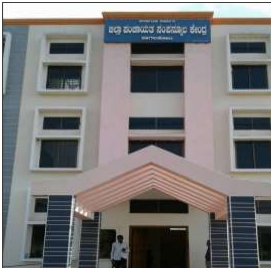
3. Construction of District Panchayat Resource (Power) Crushing Center in Navanagar
