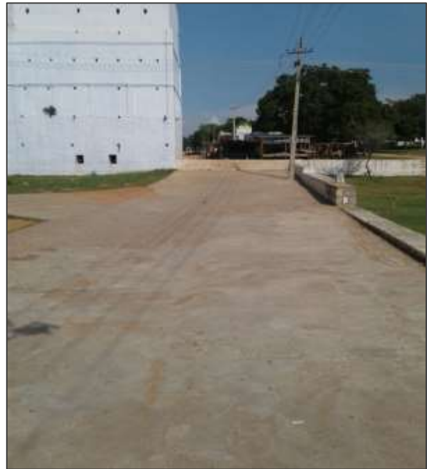
2. Construction of Pathways in front of Ameswara Temple
