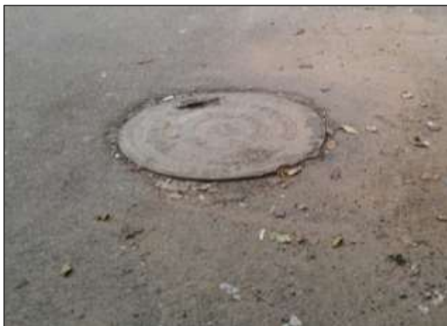
2. Old Sanitary Line and Manhole Maintenance Works of Ward No. 69
