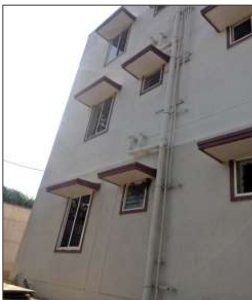
Figure 35 : External view of quarters
